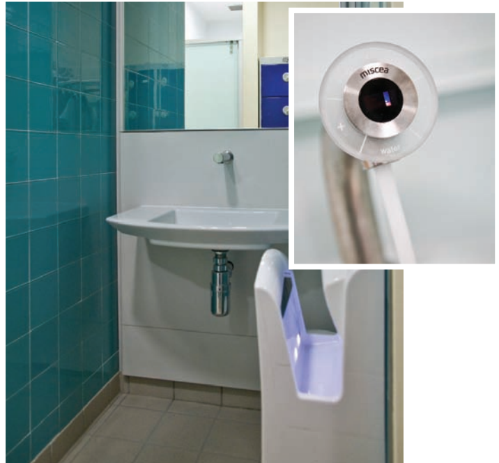
Above: The changing room
